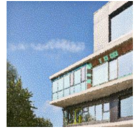
The east side of the unit "SolAce" with the green-blue glazed solar thermal collectors, on the left side on the second floor; "SolAce"东面，带蓝绿色发光的太阳能集热器，二层左面 © Roman Keller | Flickr: bit.ly/3w30xv4
